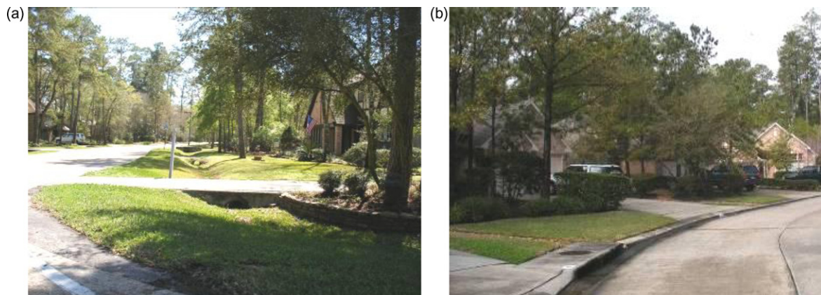
Fig. 1. Different drainage systems in The Woodlands. (a) Open surface drainage system in the first two villages. (b) Conventional underground drainage system in later villages.
