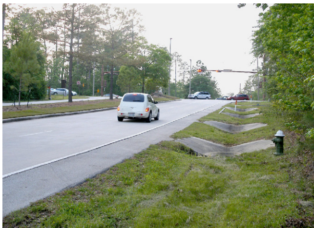
Fig. 4. Open surface drainage along collector streets. Check dams retard runoff and encourage impoundment on soils with good infiltration capacity. Also see Fig. 3.
